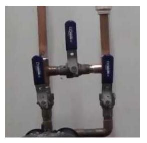
When the ball valve bypass is in service, each handle should be parallel to the plumbing or in the vertical position. To put in bypass, follow the instructions below:
